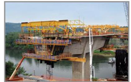
Structural concrete bridge constructions, such as this cast-in-place segmental bridge, are gaining popularity with DOTs as a way to build bridges.
