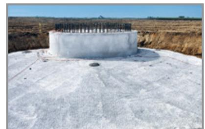
Wind turbine farms are built all over the country, with concrete playing a vital role. Foundations, such as the one shown here, use from 220 to 420 cubic yards of concrete, depending on the height of the tower.
