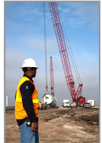
The biggest challenge on the Settlers Trail project was carrying out construction during the winter. Early spring delivery of the turbines meant that enough foundations had to be installed and backfilled so that trucks would be able to pull up to the foundation to drop off components for the cranes to pick up.
