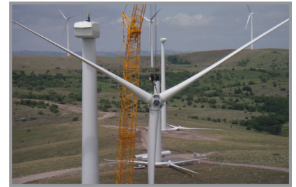
A crane maneuvers the rotor into place.
